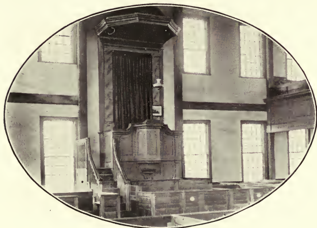
INTERIOR OF ROCKY HILL CHURCH
